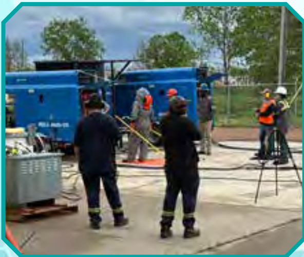
◀ Voltage Tuning of SAFER 4160V Turbine Generators
