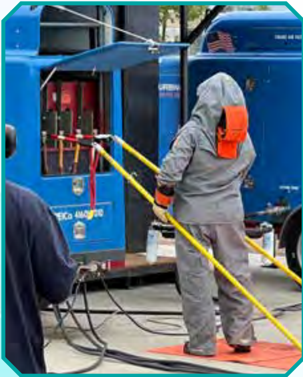
▲ Voltage Tuning of SAFER 4160V Turbine Generator
