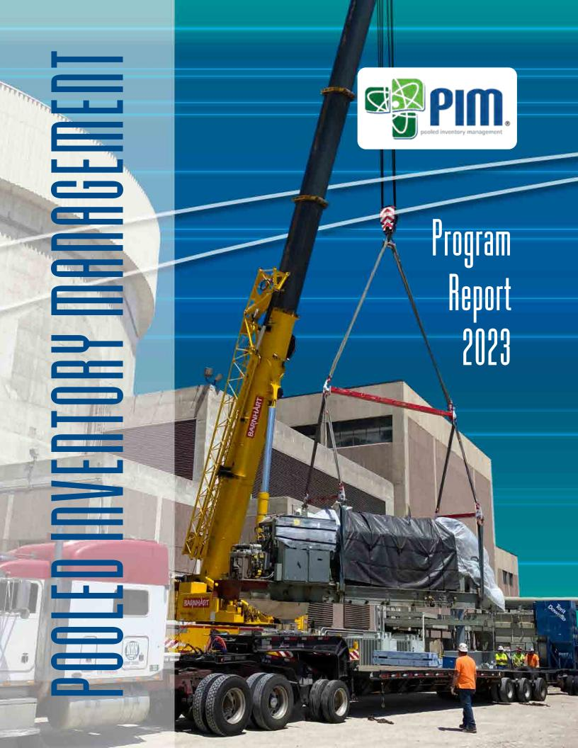
On the Cover: A Safety-Related Emergency Diesel, manufactured by EMD, is being extracted from the closed Fort Calhoun Station. Project management was performed by the PIM organization, with equipment access and movement by Barnhart Crane and Rigging. The EMD engine was purchased by PEICo as the replacement for the PIM engine that was withdrawn from the PIM inventory by Nine Mile Point 2 (NMP2) due to the catastrophic failure of NMP2's Emergency Diesel.
