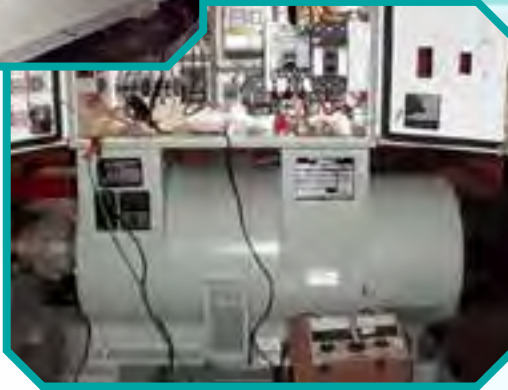
◀ Reactor Protection System (RPS) M/G Set EC Members – 3 Utilities (3 Reactor Units)
